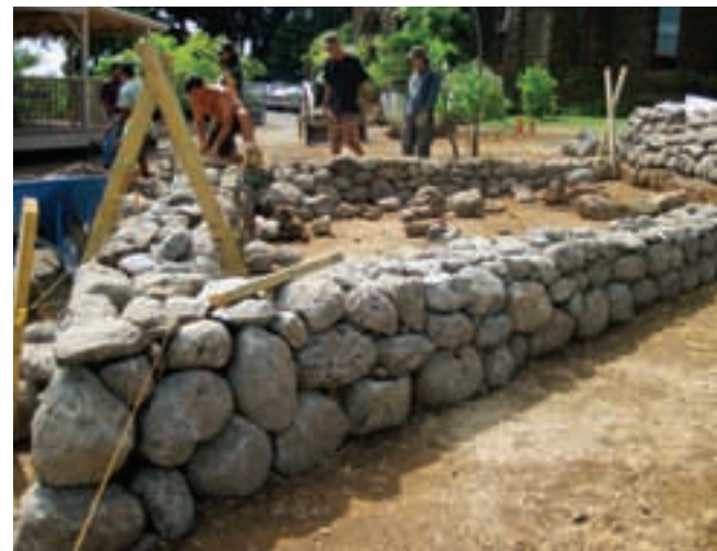
Above: Construction of the garden’s dry-stack rock walls.
